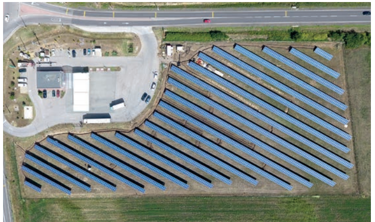
→ SOLARPARK NEWERGIES, UNGARN, 800 KWP
