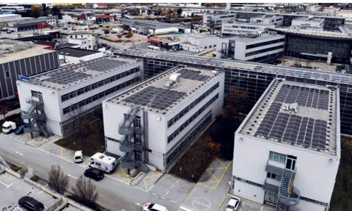
→ TECHLAB, EISENSTADT, 187 KWP
