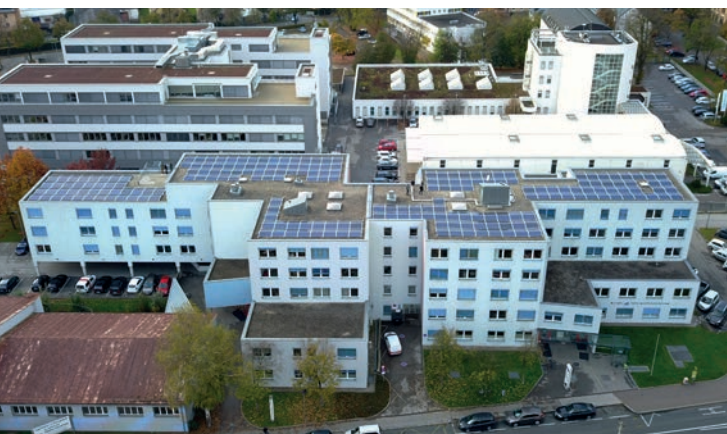
→ AMS, KLAGENFURT, 120 KWP
