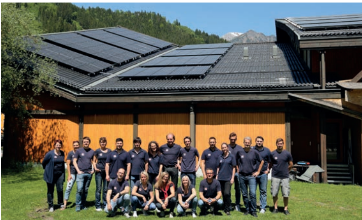
→ HOTEL ROYER, SCHLADING, 100 KWP
